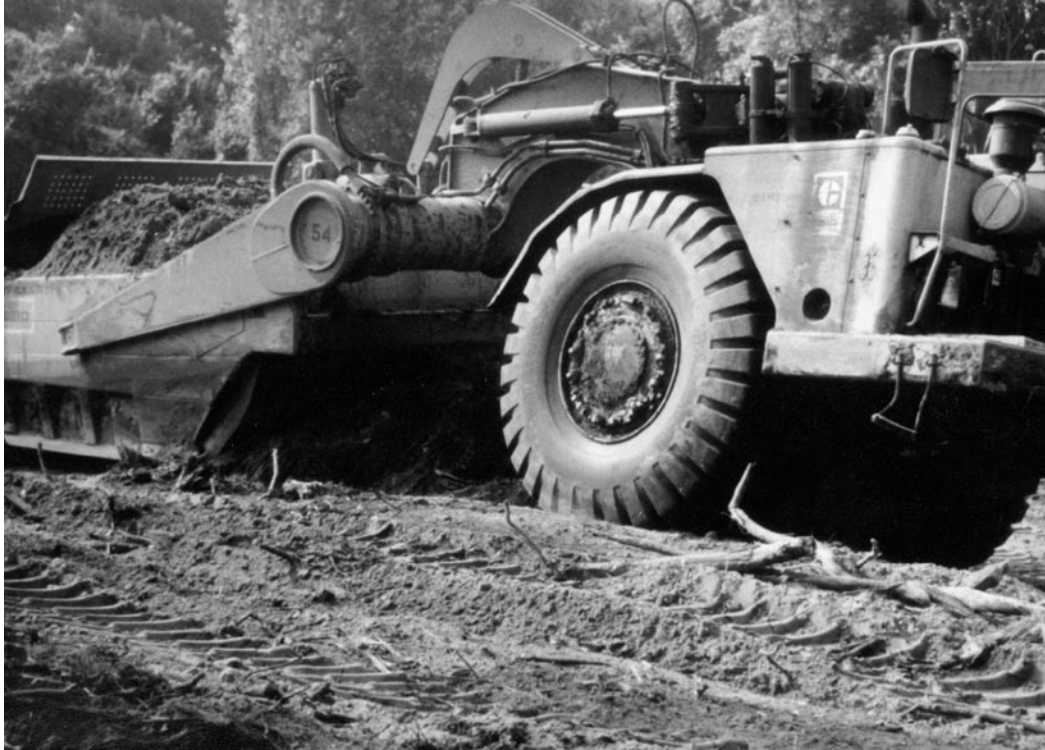
Figure 9.4. Scrapers are useful for short-distance transport of topsoil.
